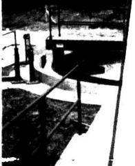
PRIMARY CLARIFIER - Jack R. Craig, superintendent of water and sewer, is standing in the background.
