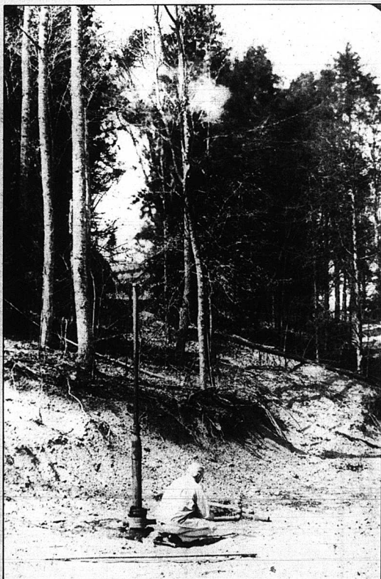
Above Leo prepares to light a second torch off his first gas well. The well which is about 2100 feet into the ground has the capacity of about 300,000 cubic feet of gas per day. In the top photo Leo smells the gas just hit on a well on Clyde Payne's property just off the Mt. Vernon by pass. Leo has leased the gas rights from Payne.
