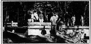
First day of cabin building
