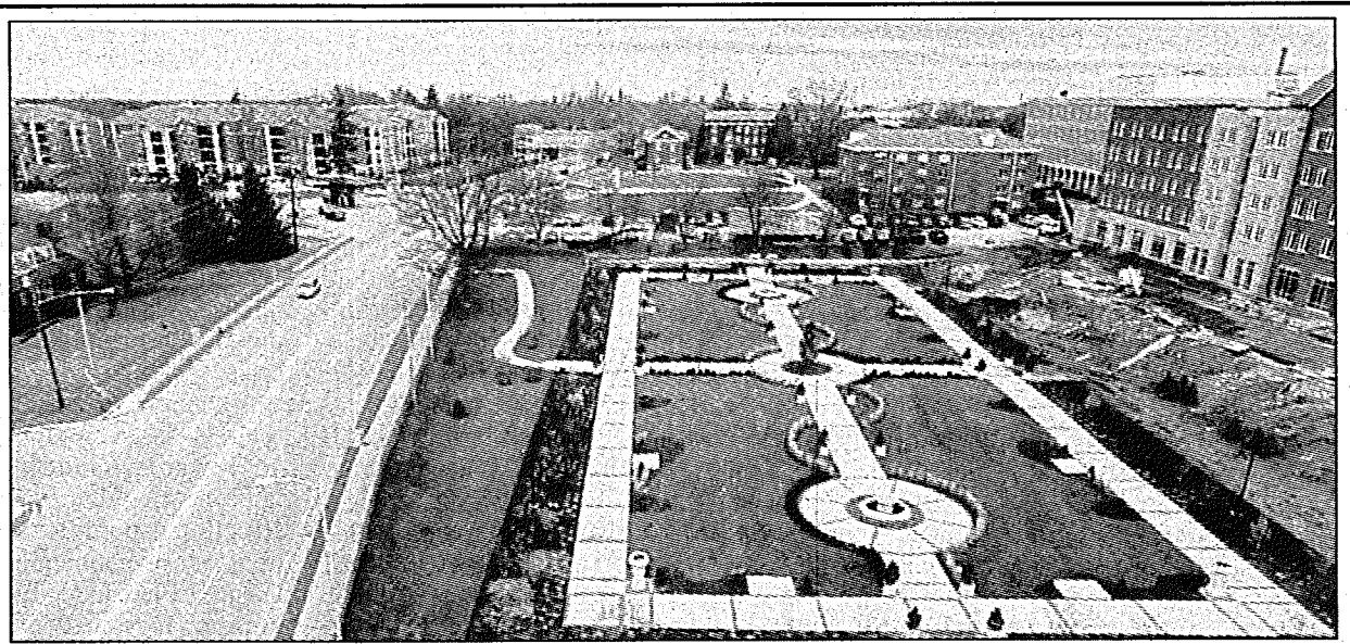
An aerial photo of Carloftis Garden from earlier this year. New Martin Hall, nearing completion of construction, is at right.
